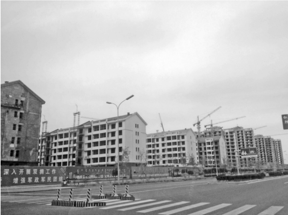
Half-finished apartment houses in Ordos. Photo by the author 2012
