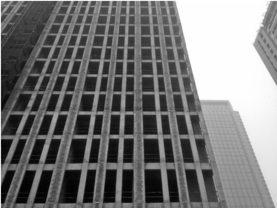
Degree of completion. Photo by J Capital 12/2/12
